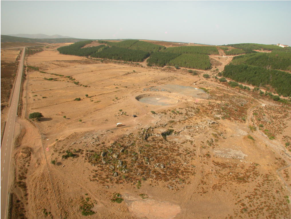
Fig. 1. This is how the Pranusanguni plateau appeared from the start of the construction activities of the base of the Sardinia Radio Telescope. An arid land, intended for sheep grazing, which will become the site of one of the main international radio telescopes.
